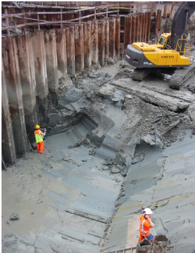
Figure 2.4 Excavation in Gothenburg clay. [27]
