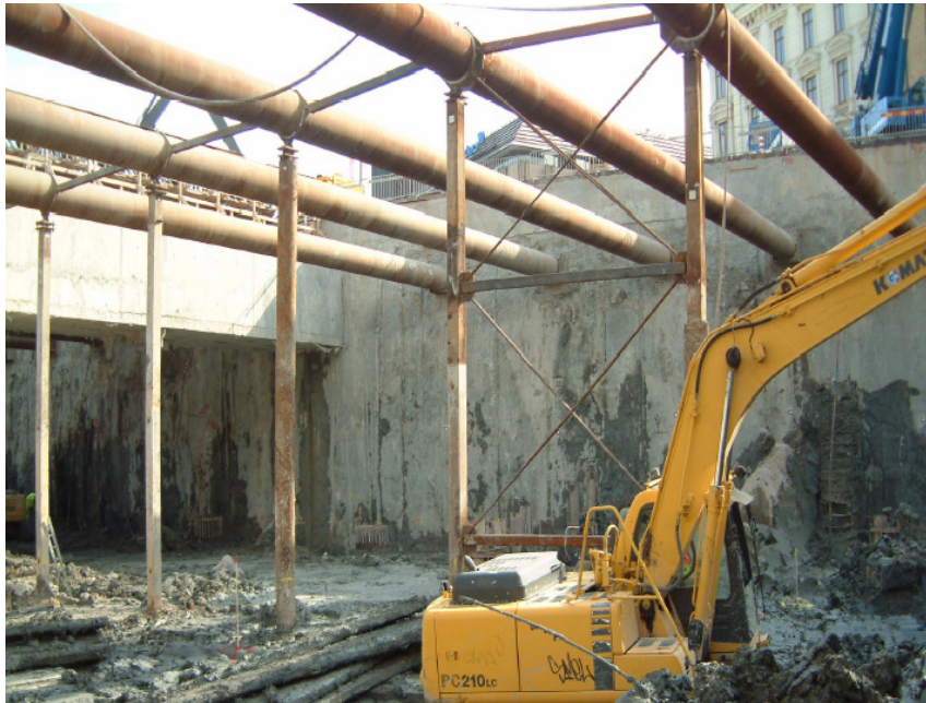
Figure 3.10 Props with vertical braces. [27]
