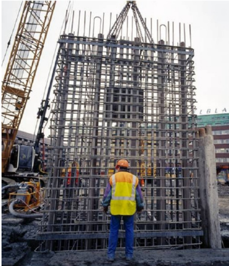
Figure 2.3 Lowering reinforcement cage into trench. [27]
