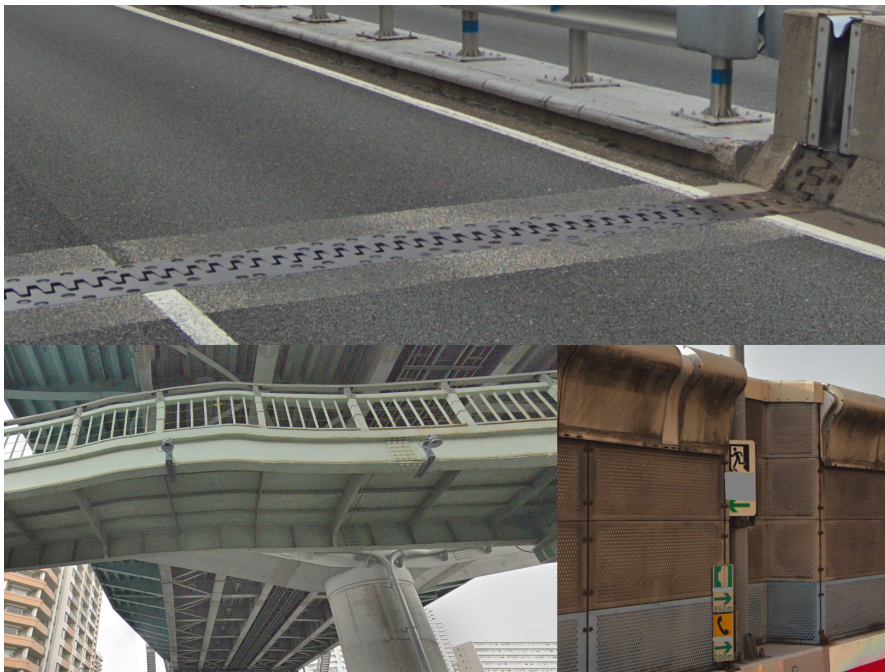
Figure 4.18: Zoomed in view of objects that might cause unwanted reflections that resulted in a false intervention. Image: partly censored screenshots of Google Street View[21].
