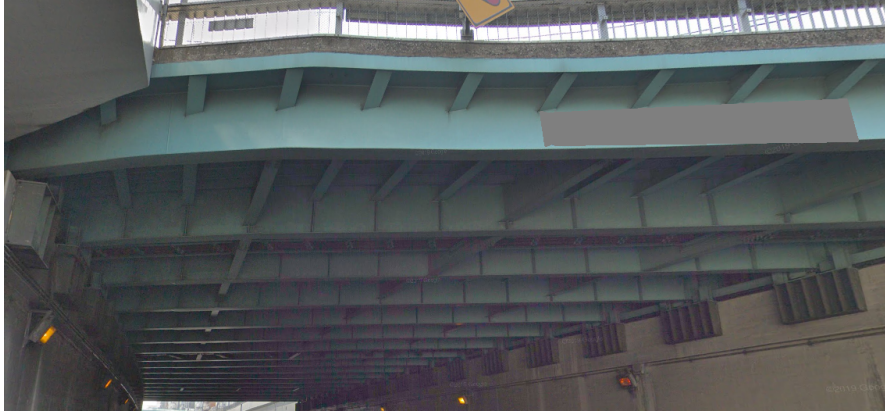
Figure 4.17: A third category of road environment where multiple false interventions have occurred. The ceiling of the tunnel has a metal grid structure which can cause many unwanted reflections. Image: partly censored screenshot of Google Street View[21].
