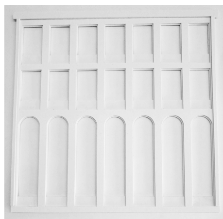
Arch spanning over two floors
