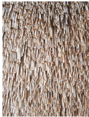
Figure 7. | Thatched facade of local reeds.
