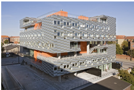
BIKUBEN KOLLEGIET Architects:AART architects Year: 2007 Location: Copenhagen, Denmark Category: Student housing Area: 7000 m 2 Units: 107 dorm rooms
