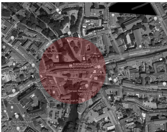
image 10 - Location of Krambrücke bridge, google image
