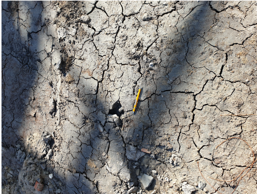
Figure 6.3: Cracks on excavation bottom in studied excavation.
