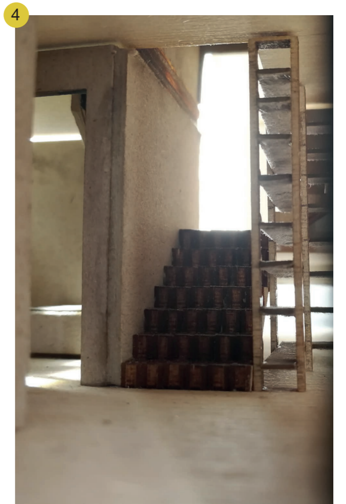
View from the entrance, looking towards the first floor bathroom and the staircase.
