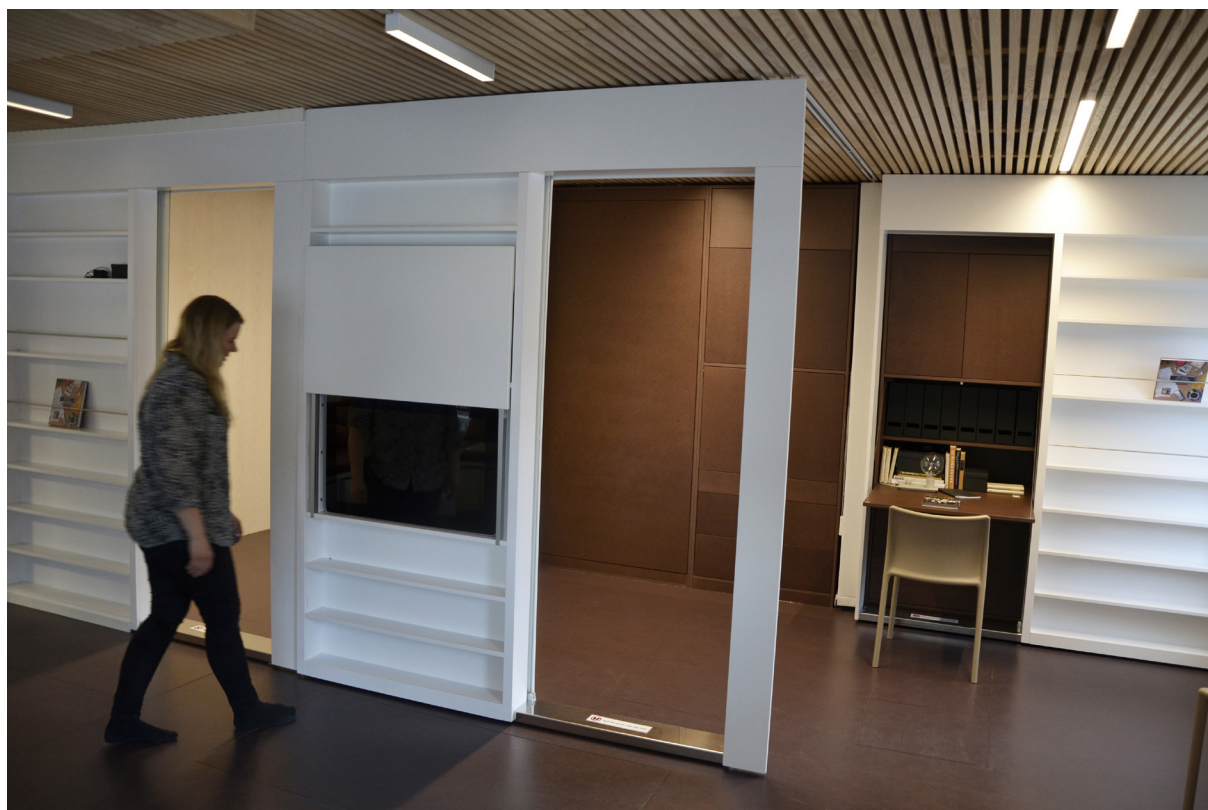
Fig. 54. Movable walls in Drömlägenheten (Own photo, 2019)
