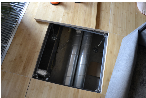
Fig. 57. Raised floor with installations beneath (Own photo, 2019).
