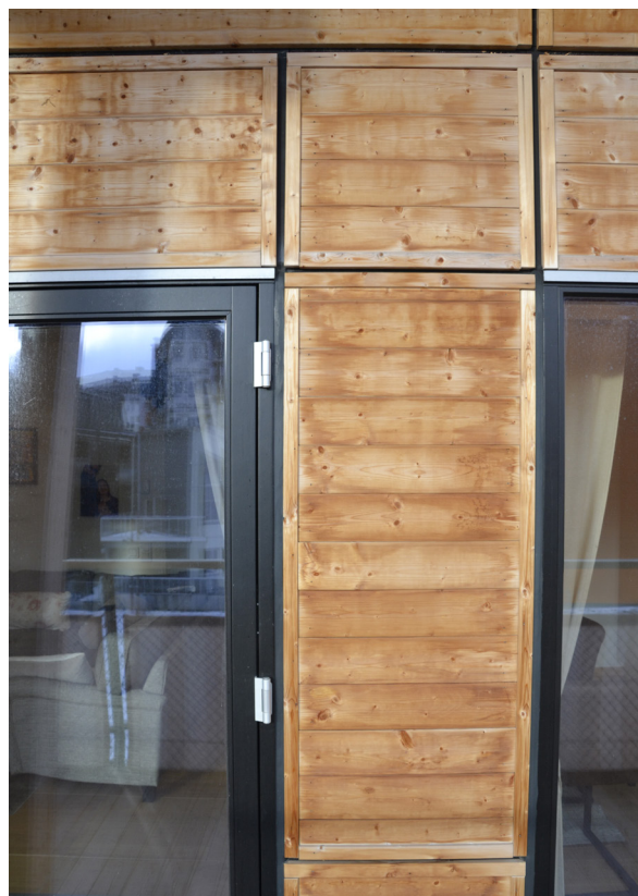
Fig. 58. Exchangeable exterior wall (Own photo, 2019).
