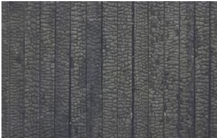
Shou shugi ban, charred facade Retrieved from textures.com
