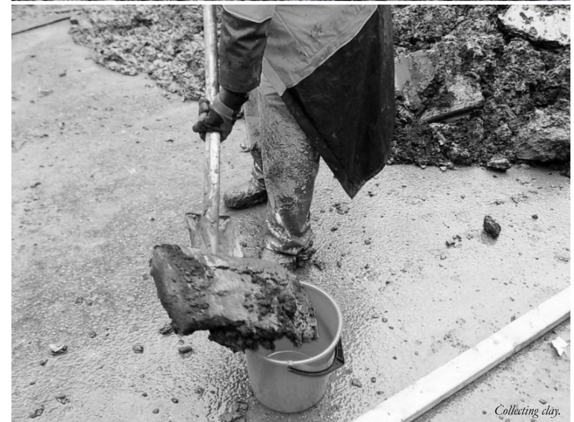
Excavation of clay in central Gothenburg.
