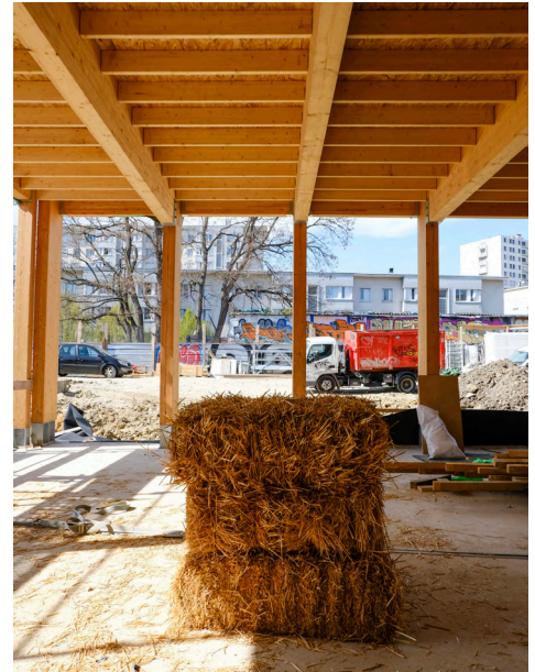
Custom ordered compact straw bales used for wall insulation from a farmer in Fontainebleau, France (70km from the construction site)
