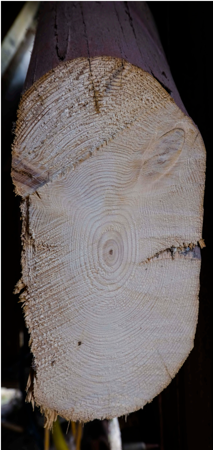
Figure 55: Section through structural timber in barn
