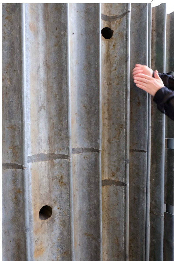
Metal roof gutters applied vertically on a wooden structure
