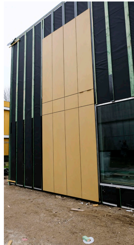
CRL exterior wall
