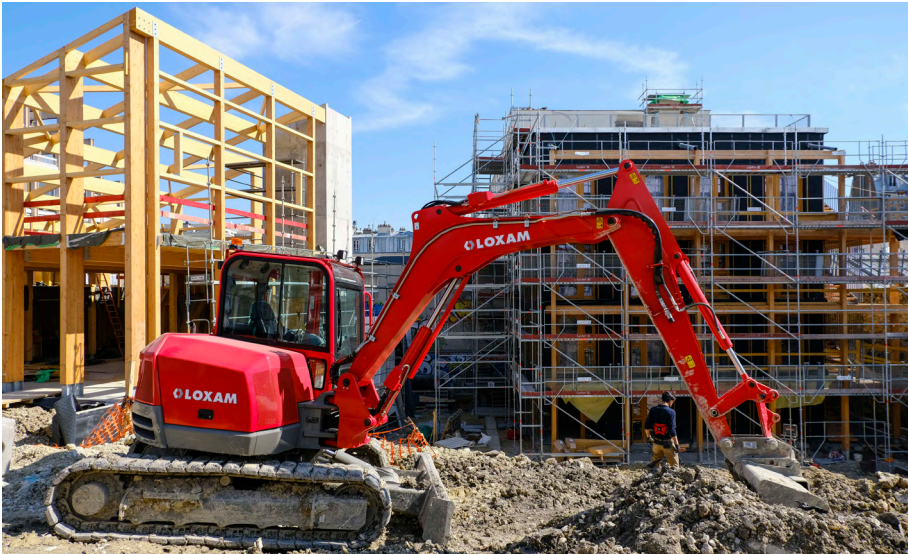
The project under construction in Paris March 2019
