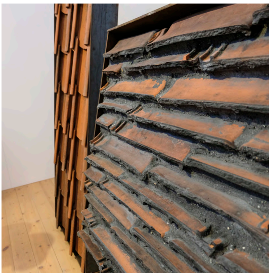
Figure 52: 2 Roof tile facades at Lendager's Wasteland Exhibit vertically hung on clips & stacked with mortar (January 2019)
