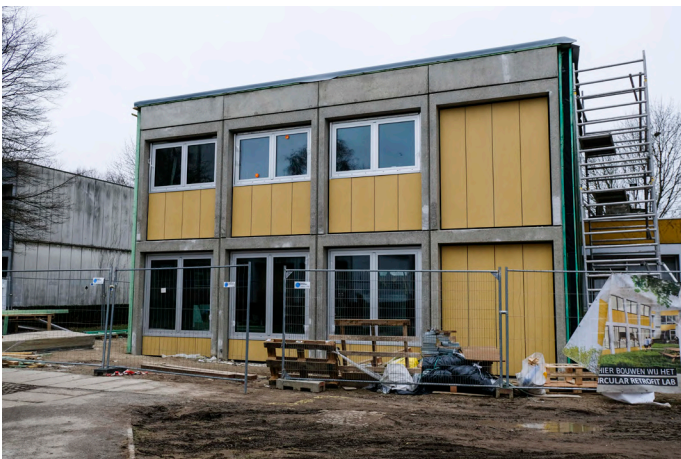
Circular Retrofit Lab under construction (February 2019)
