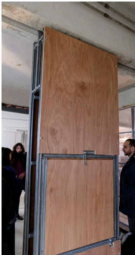
CRL interior partition using Gerberit's in-wall toilet tank system
