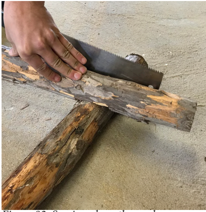
Figure 82: Sawing along the angle
