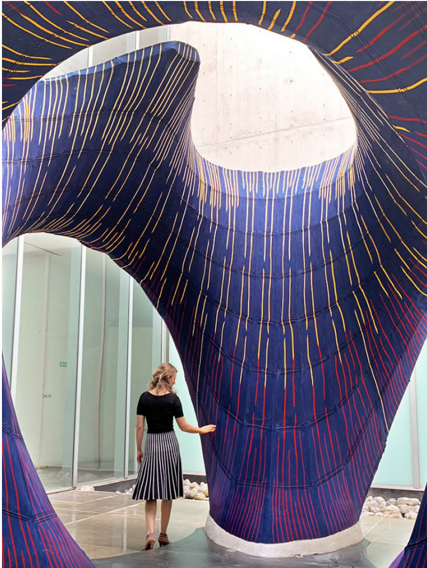
Figure 8. KnitCandela. Concrete pavillion using textile as framework. By Zaha Hadid Architects in collaboration with Block Research Group ETH Zürich. Photo: Philippe Block.
