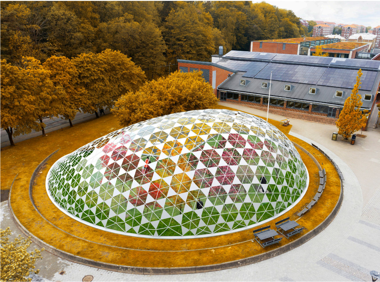
Figure 33: Illustration of a greenhouse on the Chalmers campus. A rigid shell structure with glass panels.
