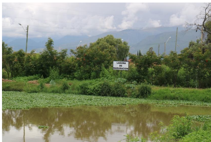
Figure 50d: Maturation pond with plants growing extensively.
