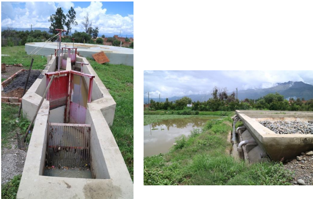
Figure 27: Treatment units at the WWTP of El Paso. Left: Primary treatment unit with screens, sedimentation channels and bypass. In the background the circular basin of the UASB reactor. Right: Secondary treatment unit consisting of two anaerobic filters (right), the outlet and the maturation pond as a tertiary treatment step (left). Author's own copyright (Photos were taken in February 2018).
