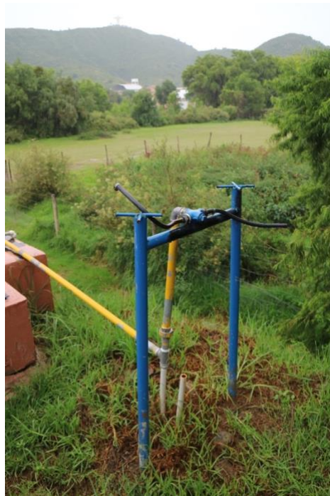
Figure 51f: Pre-treatment units, distribution chamber of UASB and rests of the gas burner that was stolen at the beginning of this year.
