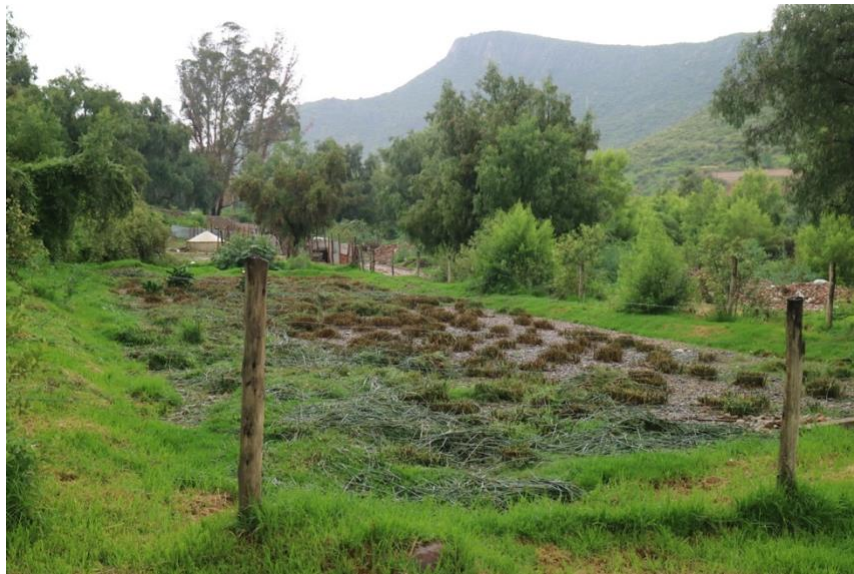
Figure 51h: Inlet to the constructed wetland (on top) and constructed wetland (on bottom).
