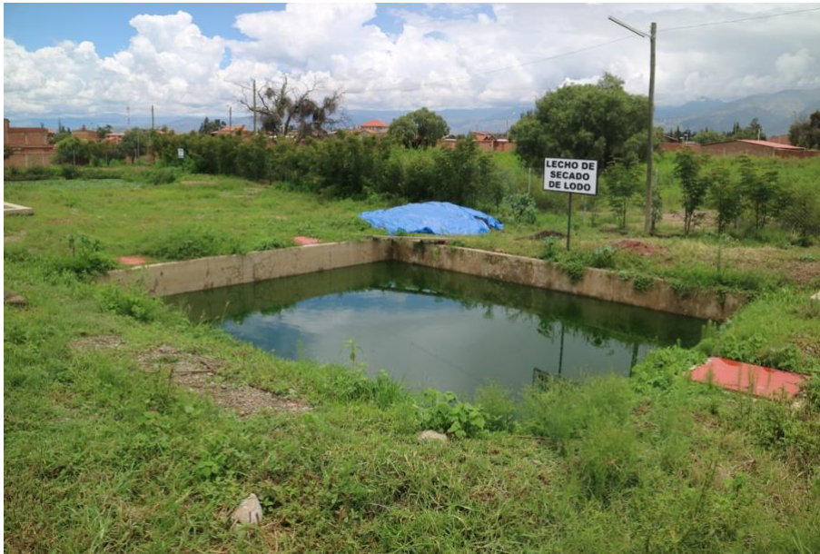
Figure 50e: Drying bed during rainy days.
