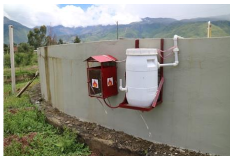
Figure 50b: UASB (on top) and gas burner (on bottom).
