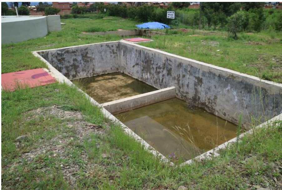
Figure 50f: New treatment unit to improve the WWTP's performance in construction.
