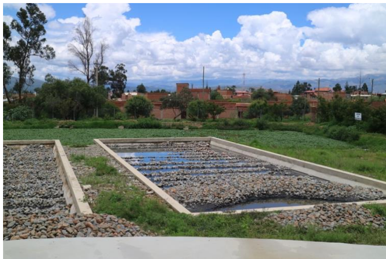
Figure 50c: Anaerobic filters. During dry days (on top) and during rainy days (on bottom).
