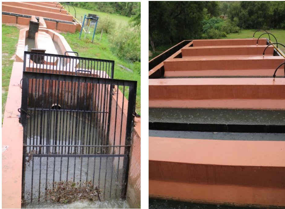
Figure 30: Primary treatment unit (left) with two screens in series, the sedimentation unit and the Parshall channel, and the UASB reactor (right) at the WWTP of San Pedro Magisterio. Authors own copyright (Photos were taken in February 2018).
