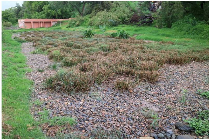
Figure 31: Drying bed, connected to the UASB reactor (on top) and planted wetland with horizontal flow (on bottom) at San Pedro Magisterio. Authors own copyright (Photo was taken in February 2018).
