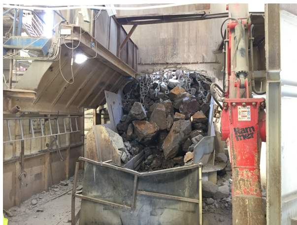
Figure 4.2: Primary crusher with feeder and rock breaker.
