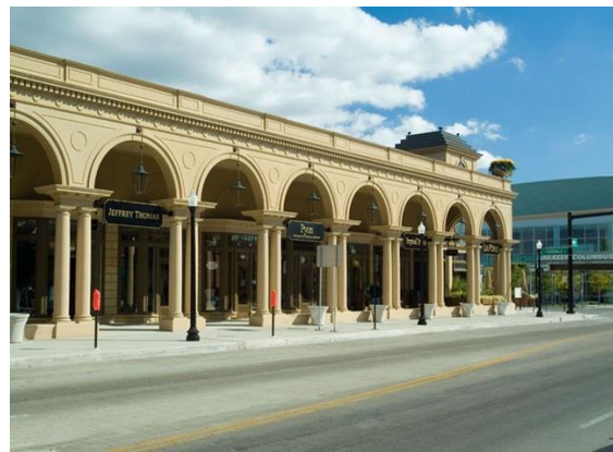
Figure 5 The Cap after being re-built. Credit to David B. Meleca Architects (2004a)
