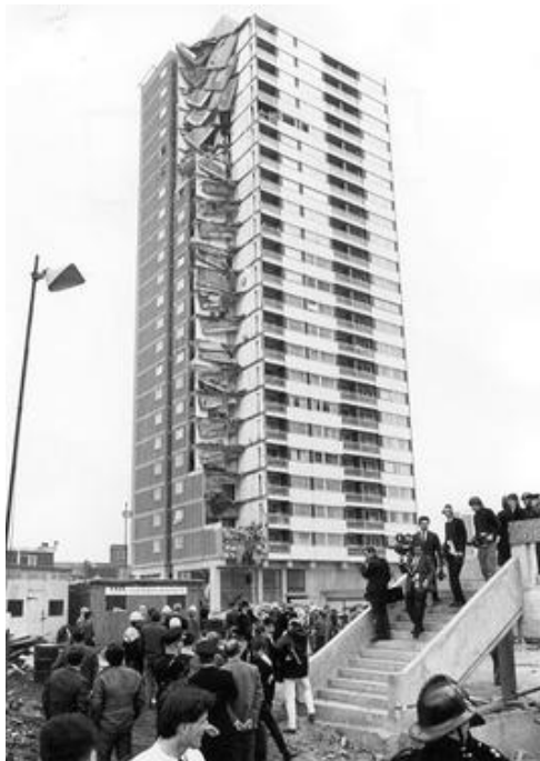
Figure 5.1 Partial collapse of the corner of Ronan Point in East London as a result of a gas explosion in 1968 (The Daily Telegraph, 1968).
