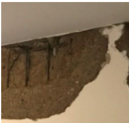
Figure 2.3 Spalling of concrete wall. Photo: Elias Fritzson. (Reproduced with permission from the photographer.)
