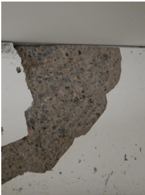
Figure 2.3 Spalling of concrete wall. Photo: Elias Fritzson. (Reproduced with permission from the photographer.)
