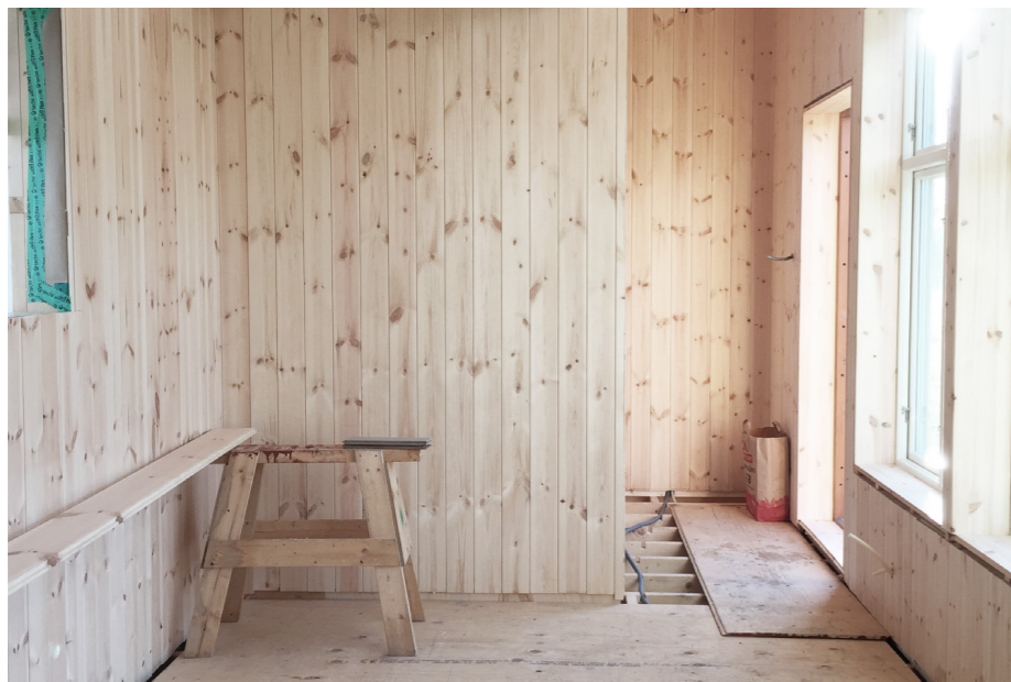
Image 11: CONSTRUCTION OF THE STANDARD HOUSE "EGNAHEMETT" (Own photo)
