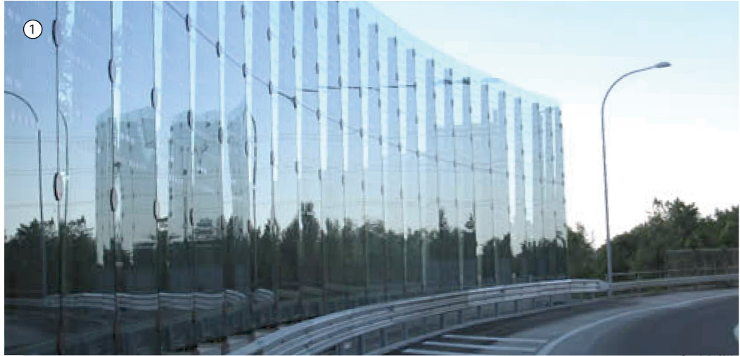
An acoustic barrier that aims to reduce the noise but still allow visual connection
