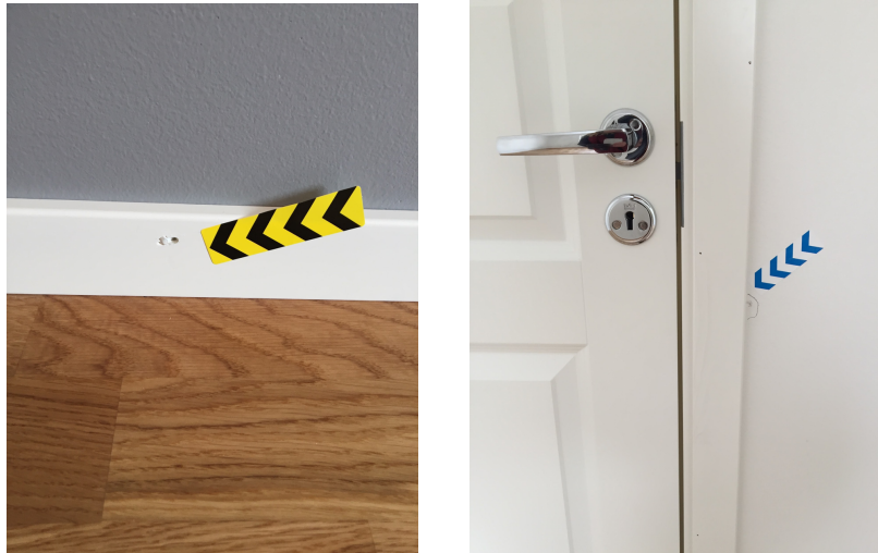
Figure 8 and 9: The black and yellow tape consider defects for the contractor, the case company. In this case the list needs to be replaced. The white and blue tape consider defects for the painter. In this case, a screw head protrudes.
