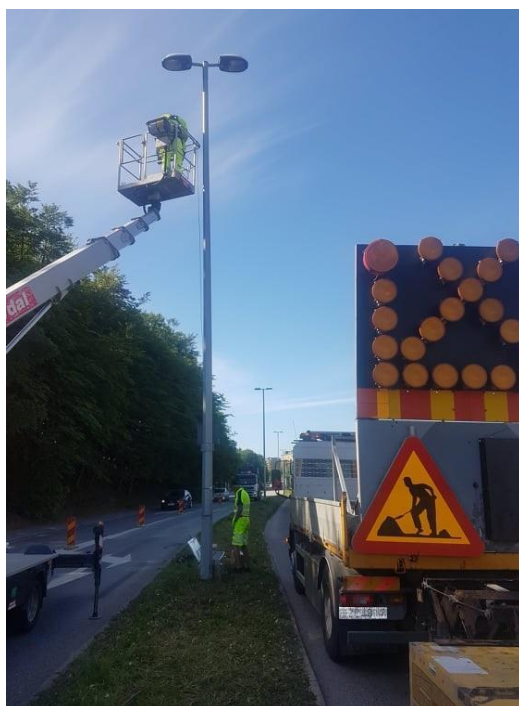
Figure 3.2 The cameras were mounted by a skylift.
