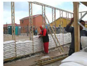
Sandbag structural wall, MMA South Africa
