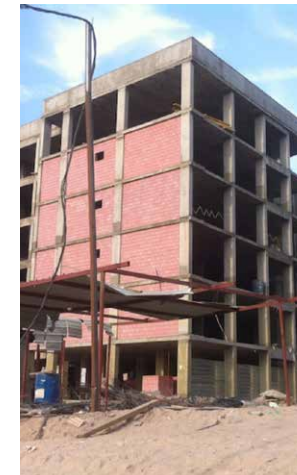
Concrete frame structure with brick wall filling, google image
