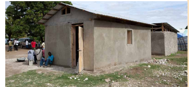
Finished gabion house prototype, haiti; Source: oxfam, 2011
