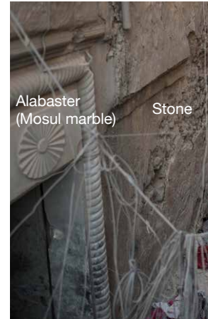
Mosul marble (Alabaster) used in entrance frame decoration.
