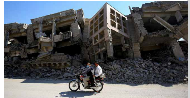
One of the demolished streetscape in Mosul, Source: Gaurdian
