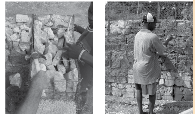
Gabion cages being filled with rubble and plastered to form a wall
