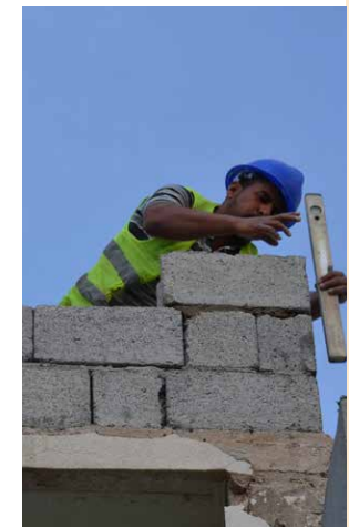
Concrete block wall structure Mosul, UNHABITAT
