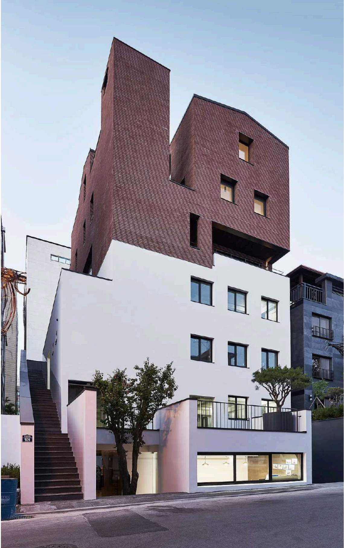
Figure 4. Sky House. (TRU Architects, 2015)
