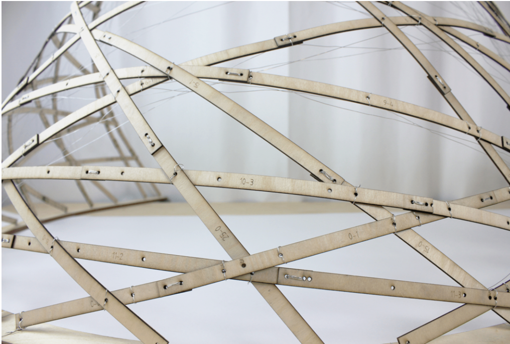
Figure 5.5: Overlap, weaving and lath coupling
