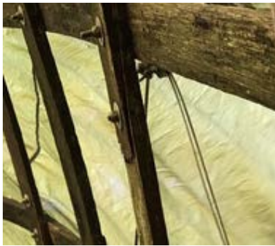
(a) Joint in Earth Center Forest Garden Grid Shell (Grant, 2017)
