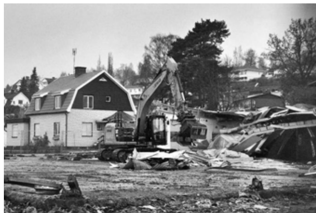
The site was bought by the municipality in 2010, and after that the demolition has been done gradually.
