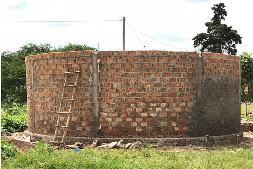
Figure 25 Picture taken in May 2018, from the construction of the new tank
