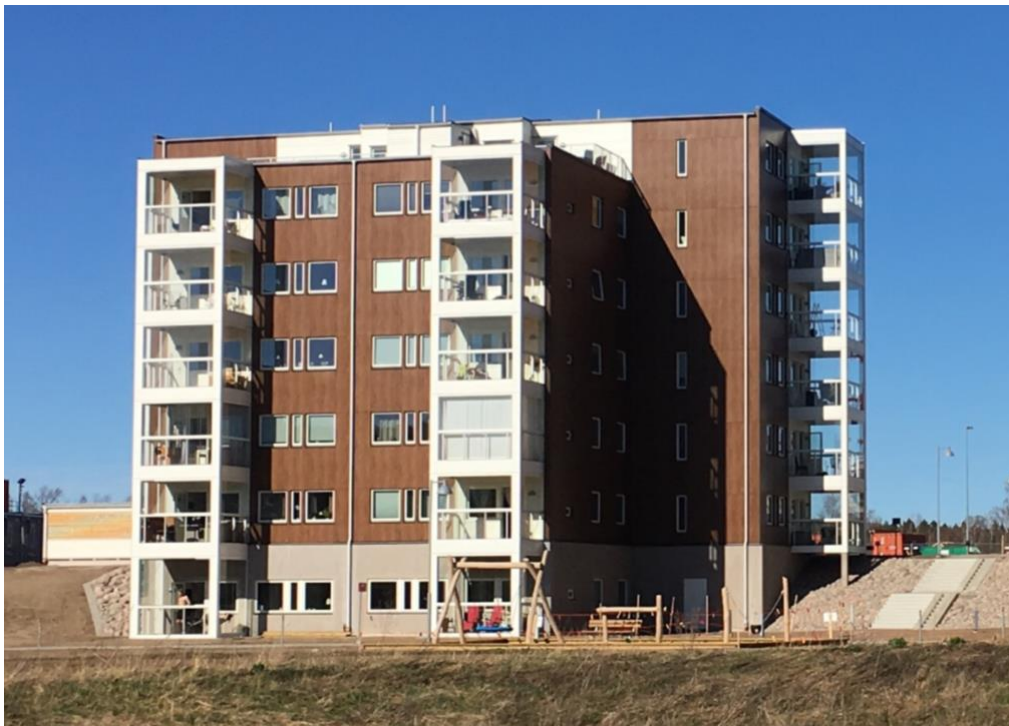
Figure 3.1 The considered building, Frostaliden 3.
