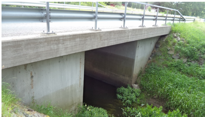
Figure 3.1 Bridge over Glasholmaån in Torsås (Trafikverket, 2018).
