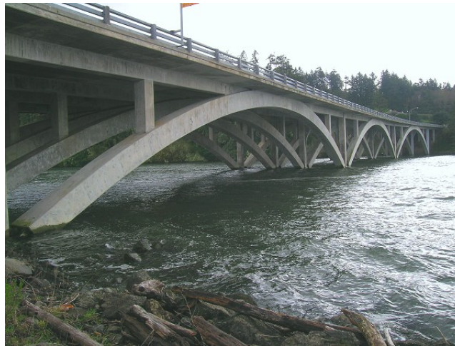
Figure 4.5 The Haynes Inlet Slough bridge in Oregon, with Alloy 2205 stainless steel bars in critical areas (Michael Goff, 2008).
