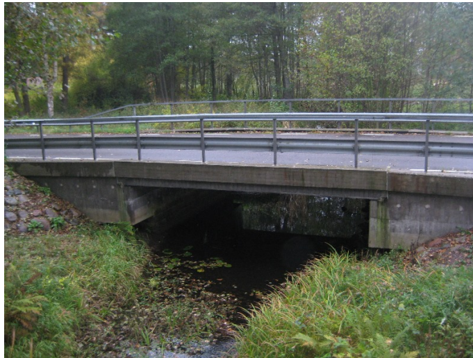
Figure 3.3 Bridge over Närvaån in Mönsterås (Trafikverket, 2018).
