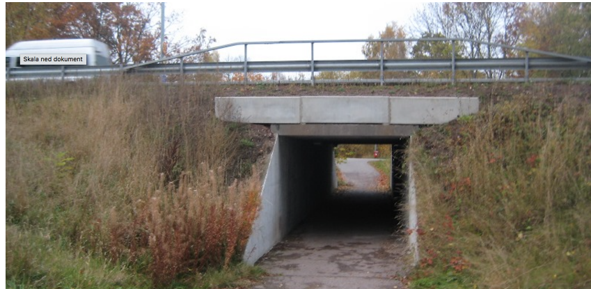
Figure 3.6 Bridge over walk- and bike path in Oskarshamn (Trafikverket, 2018).
