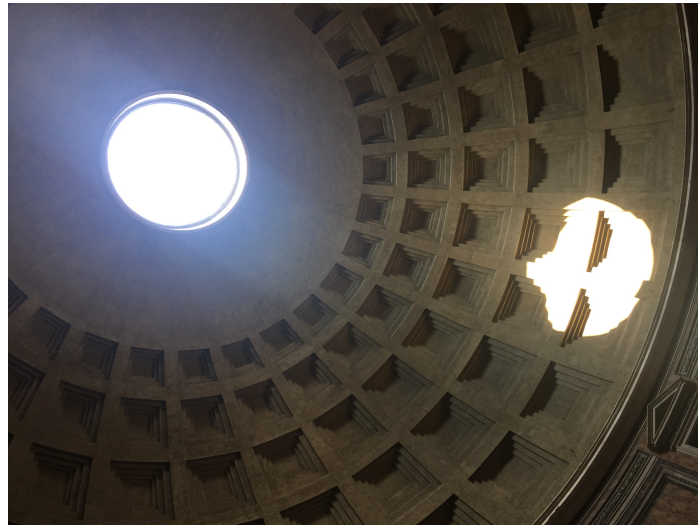
Figure 2.1 The dome of the Pantheon in Rome, unreinforced concrete structure constructed 126 AD (Dahlström, 2015).
