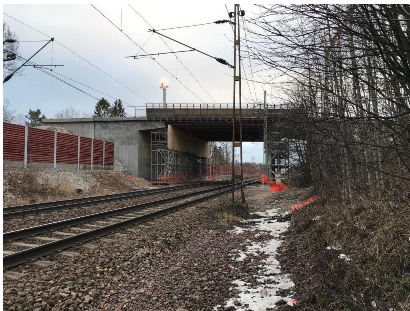
Figure 5.1 Picture of the slab-frame bridge, of which the retaining wall is a component, during construction (Trafikverket, 2018).
