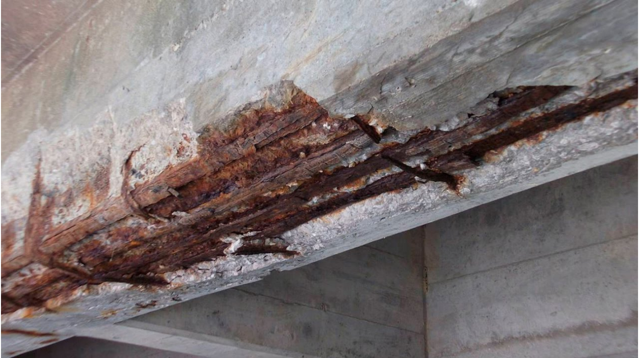
Figure 2.2 Corrosion of reinforcement in concrete, causing rust, cracking and spalling (Concrete Protection, 2017).
