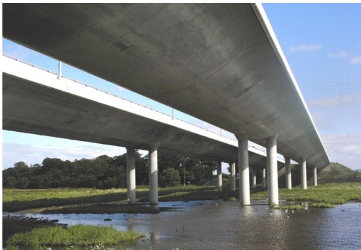
Figure 4.2 Broadmeadow bridge in Ireland, with pier stems and columns reinforced with stainless steel rebars (CBDG, n.d).
