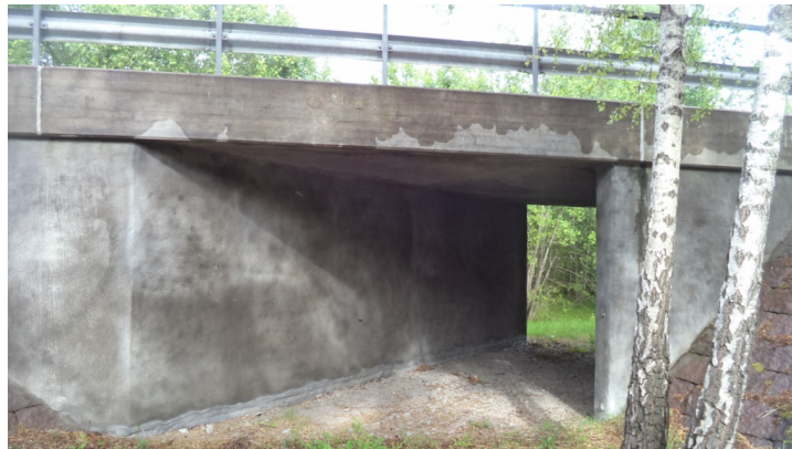
Figure 3.2 Bridge over railway track in Oskarshamn (Trafikverket, 2018).
