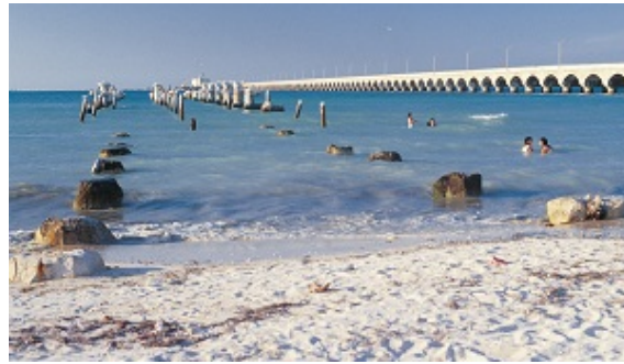
Figure 2.3 The remains of the 1972 carbon steel reinforced pier next to Progreso pier constructed with stainless steel in 1941 (Nickel Institute, 2018).
