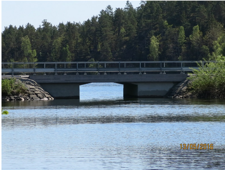
Figure 3.4 Bridge over strait in Västervik (Trafikverket, 2018).
