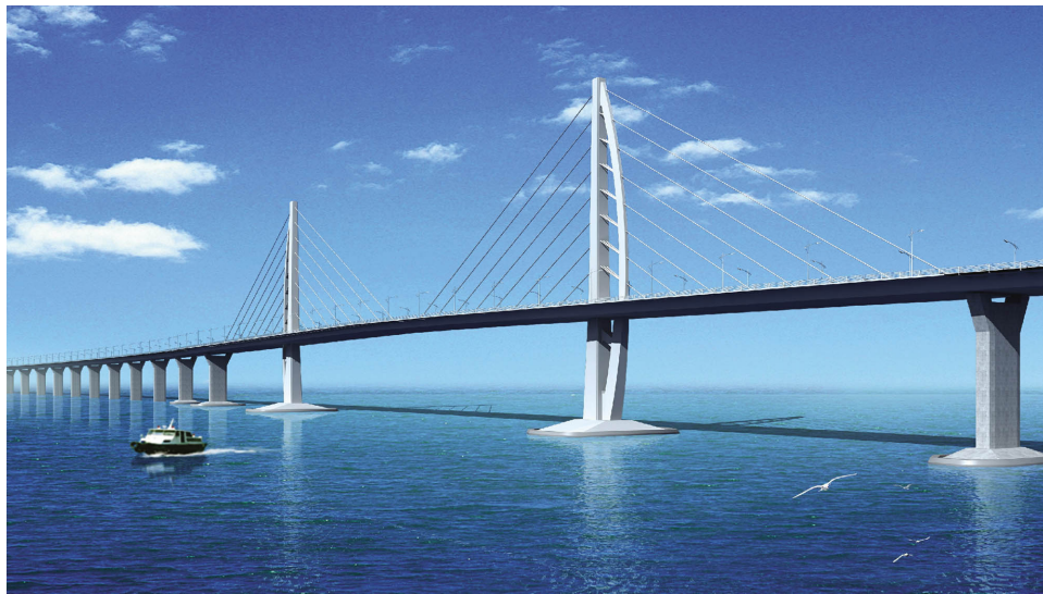
Figure 4.3 The Hong Kong-Zhuhai-Macau Bridge which connects Hong Kong with Zhuhai and Macau and is constructed with stainless steel reinforcement (© Arup, 2018).
