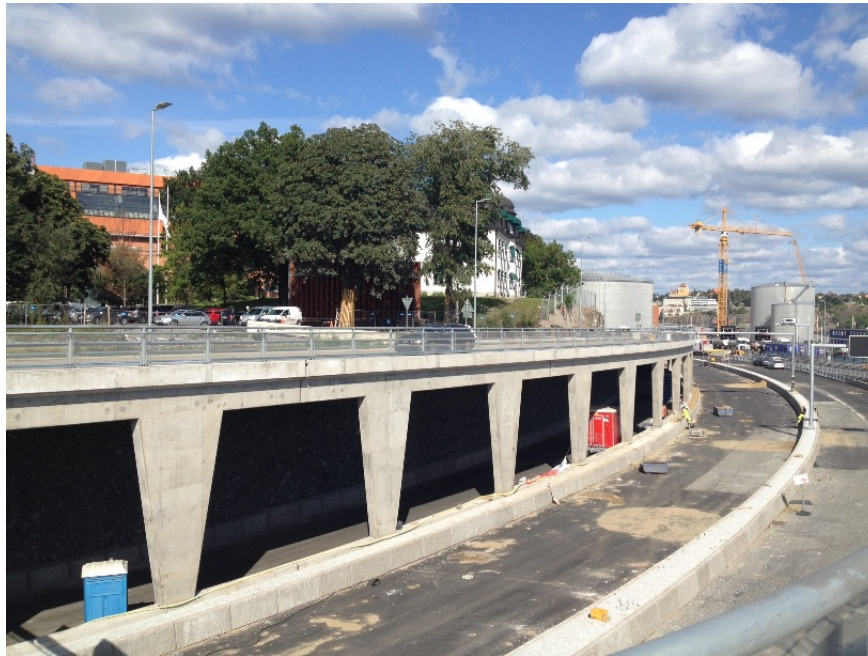
Figure 4.1 The Värtan junction in Stockholm, using lean duplex EN 1.4162 (Trafikverket, 2014).
