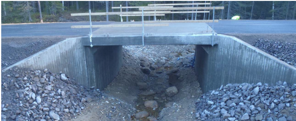
Figure 5.5 Picture of the slab-frame bridge during construction (Trafikverket, 2018).
