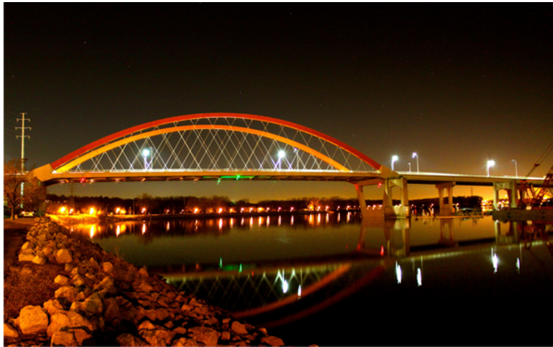
Figure 4.4 The new Hastings bridge in Minnesota, using stainless steel rebars in critical areas (MnDOT, 2018).
