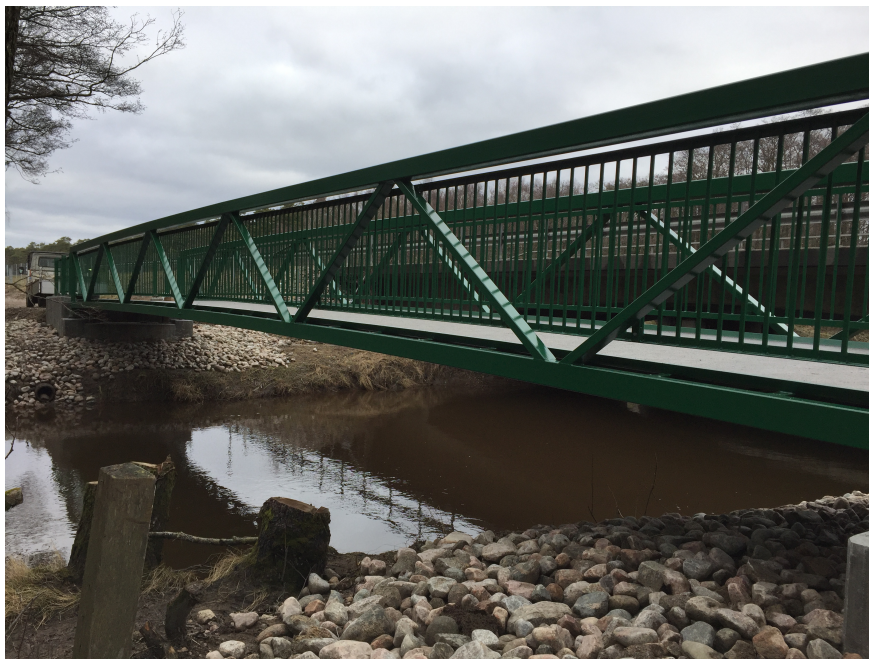
Figure 4.1: Reference project over the stream Genevadsån, picture from Ramböll (2018).
