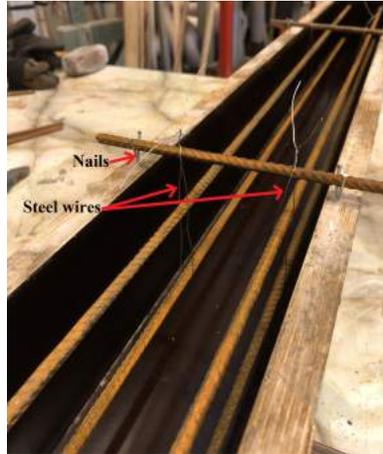
Figure 6.2 Picture showing how the bottom reinforcement were hung up.
