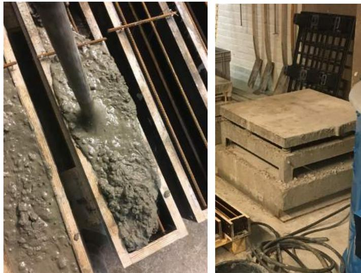
(a) Vibrating rod (Batch 1).
