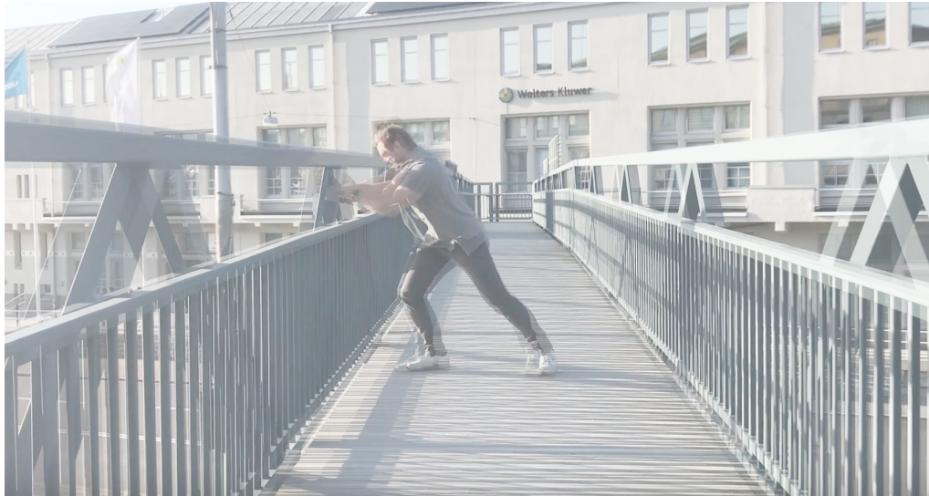
Figure 4.9: Erik Johannesson's Footbridge being put into resonance by the actions of one person. The significant lateral displacements can be seen looking at the webs.
