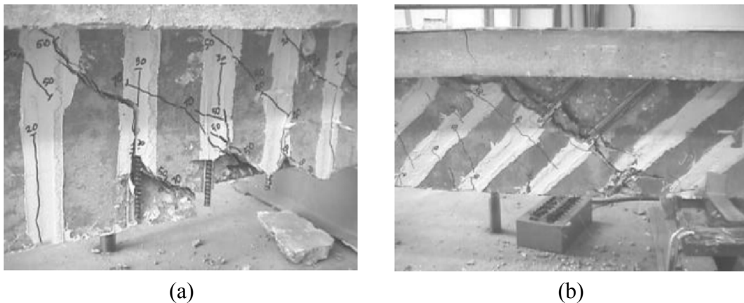
Figure 3.14 Two of the beams, after failure, studied by De Lorenzis & Nanni (2001): (a) Vertically installed FRP rods; (b) FRP rods installed with an inclination (De Lorenzis & Nanni, 2001).
