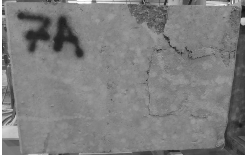
Figure 8.16 The side with recess, of Test 7 after performed structural test. The steel beam where the load was applied, is to the right.
