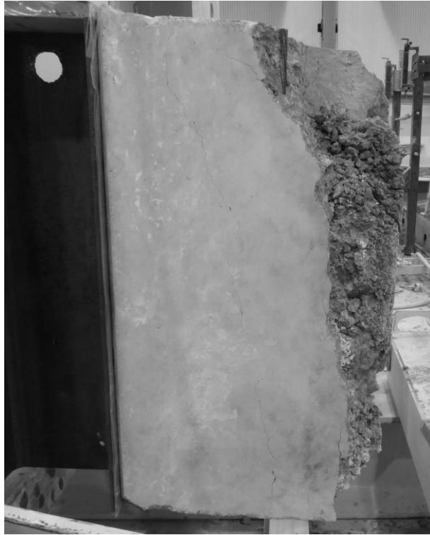
Figure 8.13 The side without recess, of Test 6 after performed structural test. Due to an abrupt failure, only the remaining concrete part, attached to the steel beam, can be seen. The steel beam where the load was applied, is to the left.
