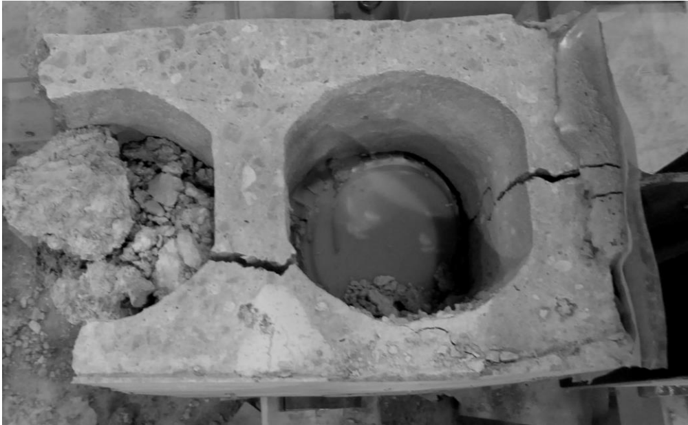
Figure 8.18 The cross-section of Test 4. This represents the general behaviour of the crack formations in all structural tests. The steel beam where the load was applied, is to the right.
