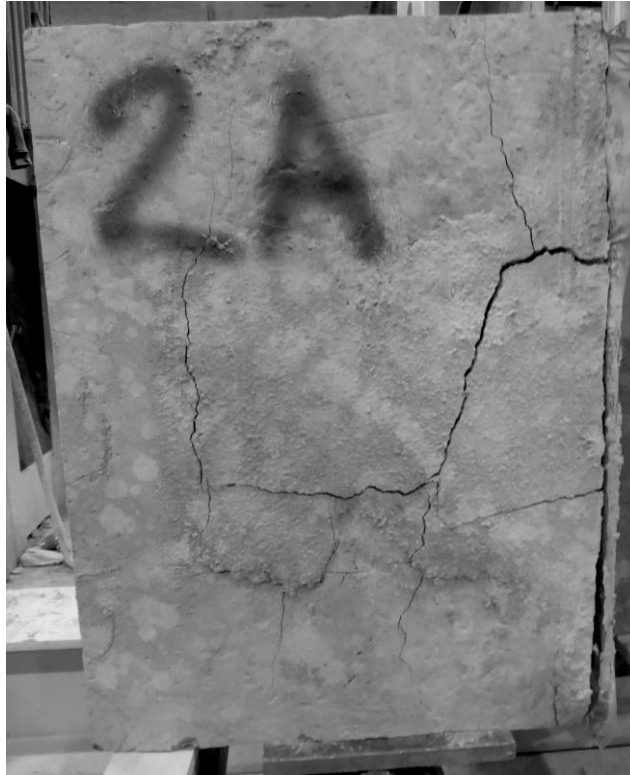
Figure 8.1 The side with recess, of Test 2 after performed structural test. The steel beam where the load was applied, is to the right.
