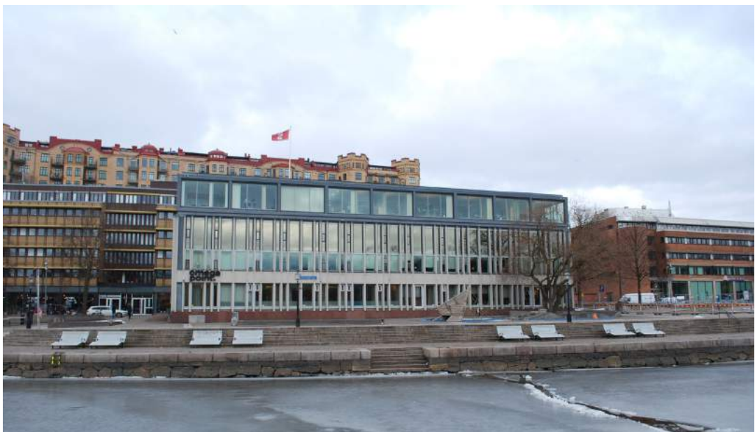
Figure 21. Office building on other side of the moat. Employs a filigree construction that is made visible as facade expression.
