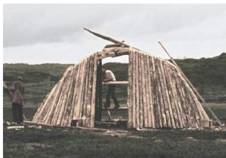
Figure 40. Construction of a Sami cot in the summer settlement Arasluokta, Padjelanta National Park. (Manske, 1982). Public domain.
