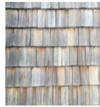
Figure 112. Wood Shingles. Author's own copyright.
