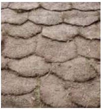
Figure 109. Peat roof placement.
