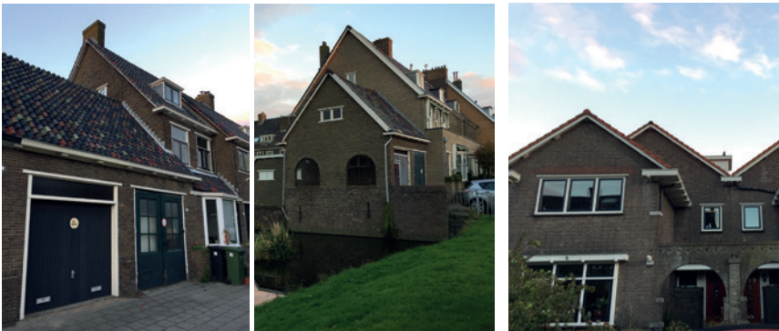
Overlapped saddle roof.
