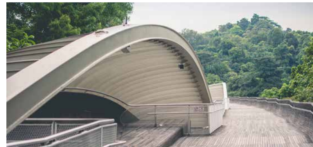
Henderson Waves, RSP Architects Planners & Engineers
