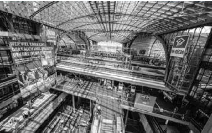
BERLIN HAUPTBANHOF STATION GMP (1993-2006)
