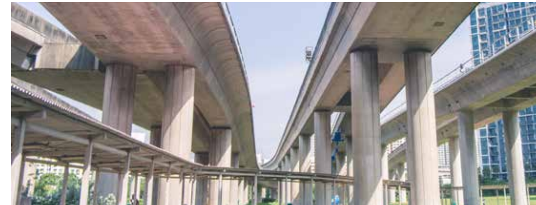
Elevated MRT rails
