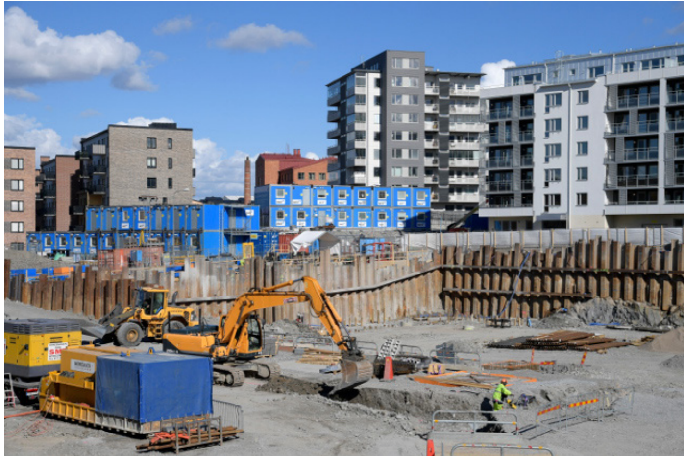
Figure 6. New apartments being built in northern Stockholm. (Anders Wiklund/TT)
