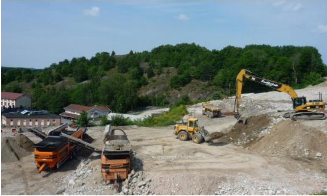
Figure 2. Excavation and soil sieving at Hexion site in Mölndal, Sweden. Photo: Åsa Landström (Landström & Östlund, 2011)
