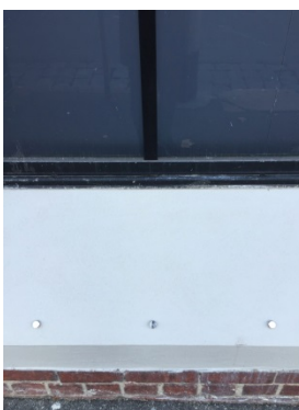
The metal pins on the bottom are skate stoppers. They are meant to stop skateboarders from grinding (Melbourne, Australia).
