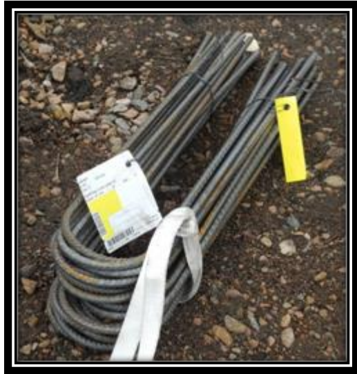
Figure 10 Reinforcement is delivered colure coded Celsa Steelservice, (2012).
