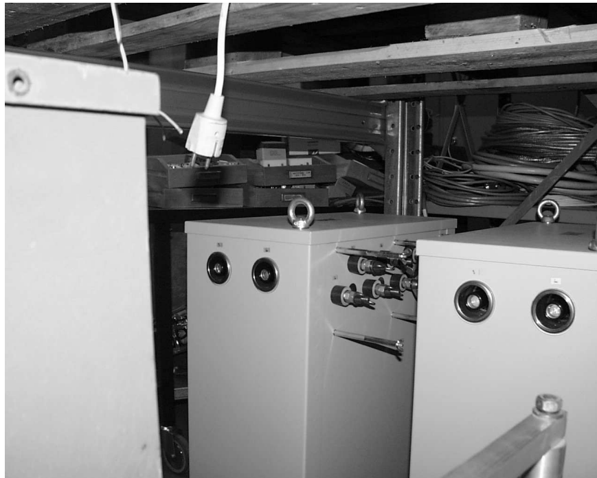
Figure 6.3: The photo show the auto-transformers. The 200A input connections can be noted on the short side of the auto-transformers and the different levels of out-put voltage can be noted on the front side on the autotransformer in the middle of the picture.
