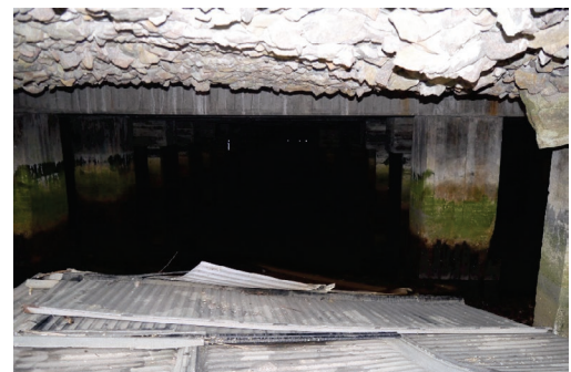
Figure 58: Photo showing the space filled with sea water under the building shown on the photo to the left.
