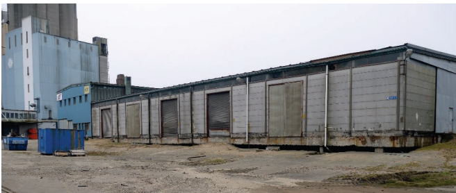
Figure 57: This photo shows the lowest point in the western part of the site. It is just about half a meter above sea level and are regularly flooded. A height difference between the foundation of the building and the ground level can be seen. Underneath this building the landfill has been washed away, shown in the photo to the right. In the background to the left, the silo building is visible.
