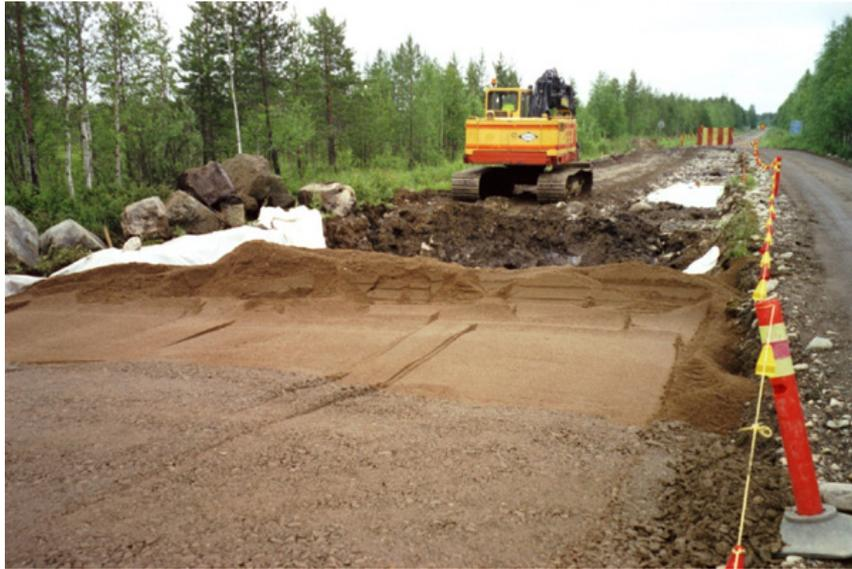
Figure 3.23: Soil replacement in road construction [83].
