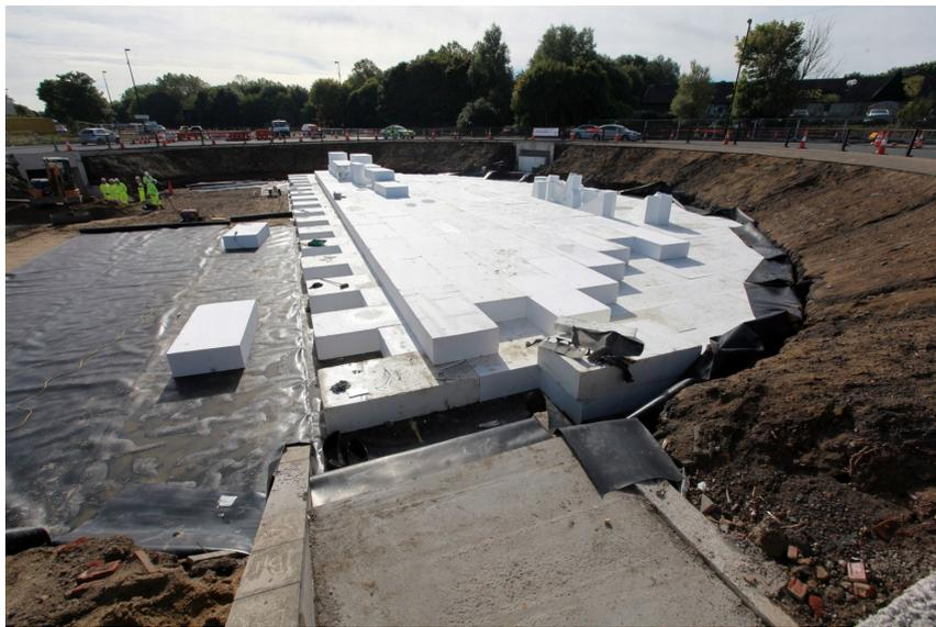
Figure 3.31: EPS as a light fill material at the Cowgate roundabout construction, Newcastle upon Tyne [104].
