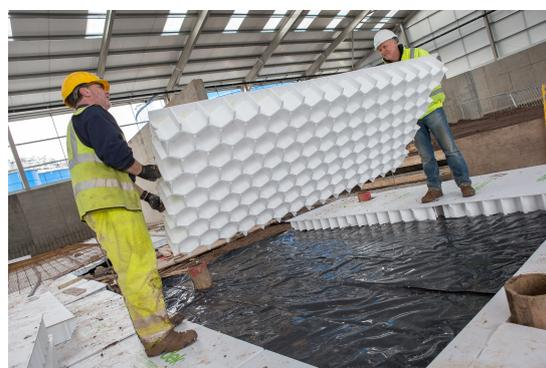
Figure 3.27: Cellcore installation under the raft [93].
