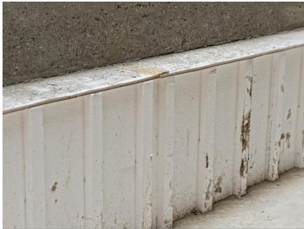
The Cellcore HG range of collapsible products has been designed to protect foundations from the effect of ground heave.
