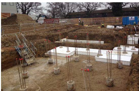
Figure 3.26: Cellcore installation around piles for the raft construction [92].
