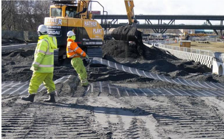
Figure 3.28: PFA with reinforcement mesh used for the road construction on the soft ground [97].
