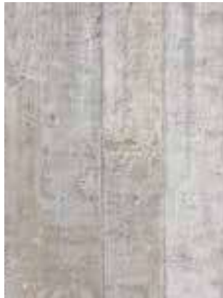
Structural surface Caste in a wooden mould 10 year old
