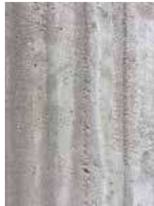
Smoother surface Caste in a plywood construction mould 10 year old
