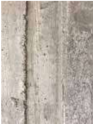
Heavily structural surface Caste in a wooden board mould 15 year old
