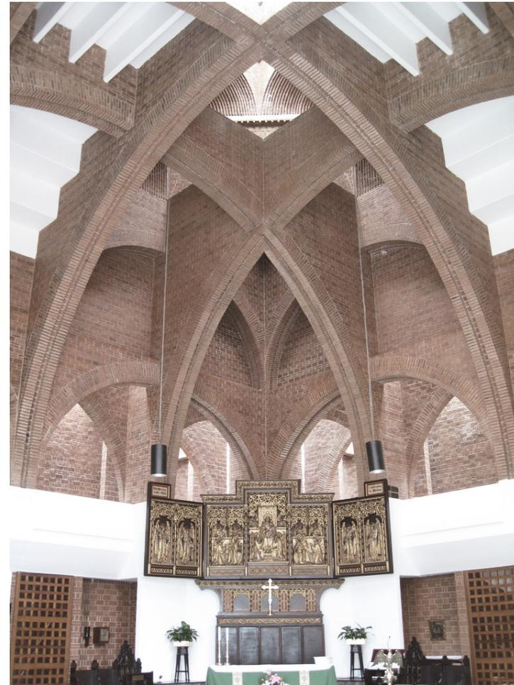
Interior scene of christ church shows that it is a structure dominate space. The double arches cross with each other and sketch the outline of interior space. Half arches hold the main structure and diffuse the daylight.
