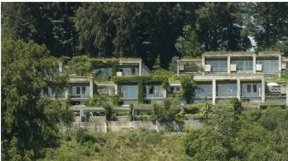
FIGURE 10 Halen housing complex by Atelier 5. Picture credit: Wikimedia commons
