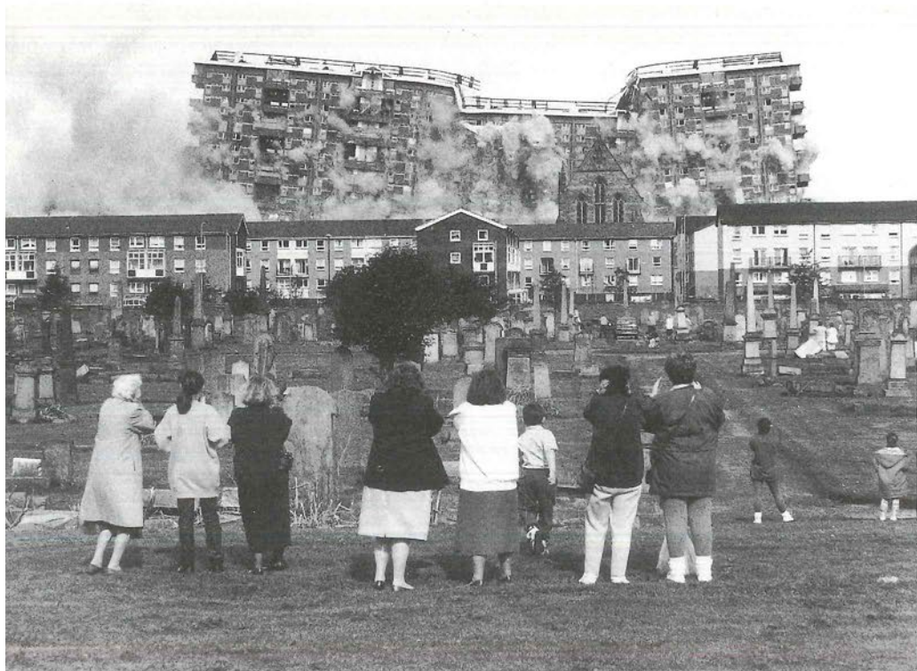
FIGURE 1 European post war development is haunted by stigma and alienation but also technical difficulties. When repairs can no longer be made, and is no longer wanted, drastical structural changes has to be made. (Mills 1994 p.145)
