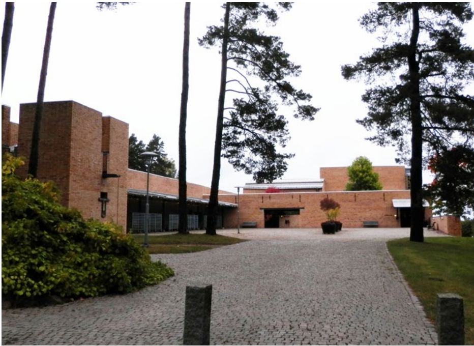
FIGURE 2 Lilla aska crematorium by Ove Hidemark. Built with soft mortar and thick massive brick walls. Photo credit: Wikimedia commons
