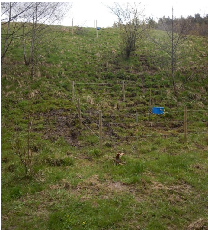
Figure 4-25. Photo taken from the bottom of Slope 2. Station Toe is closest in the photo and station Middle is seen further up in the slope. Some erosion of material in the slope can also be observed.
