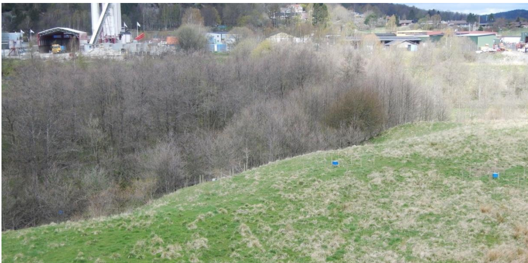
Figure 4-22. Photo taken on the Lärje River, direction north from Slope 1. It can be seen that the sides of the river channel are steep, approx. 2 meters high when the water level is as low as in the photo. Erosion protection (coarse material) can be seen near the shore to the right in the photo.
