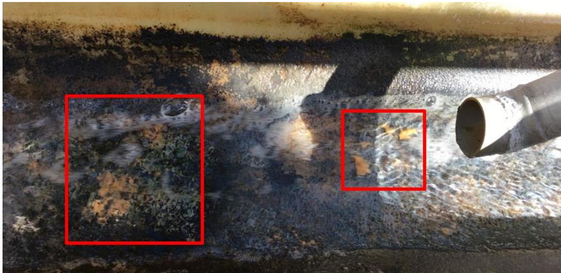
Figure 3. The growth found at the pipe inlet from the pump pit at the CRV. The growth has both an orange and a greenish tint and has been marked with red squares. The picture is taken from above.
